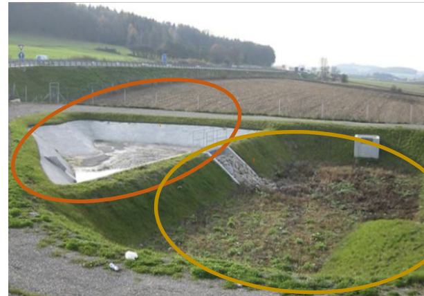
Basin combining sedimentation and infiltration
